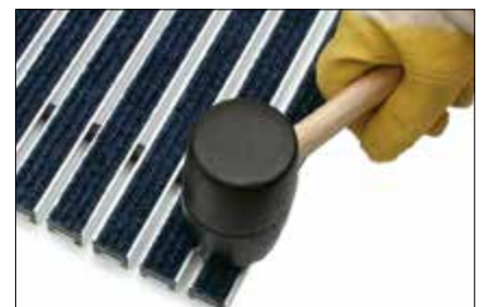
3. Place new insert into the aluminium profile using self-adhesive tape; use a rubber hammer if necessary to affix insert.
